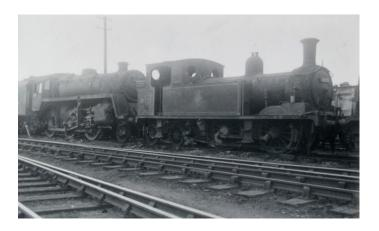
The freight allocation at this large running shed was made up by quantities of more modern machines; Southern class Q and Q1 0-6-0s, and a trio of BR 9F 2-10-0s in gleaming black livery.
