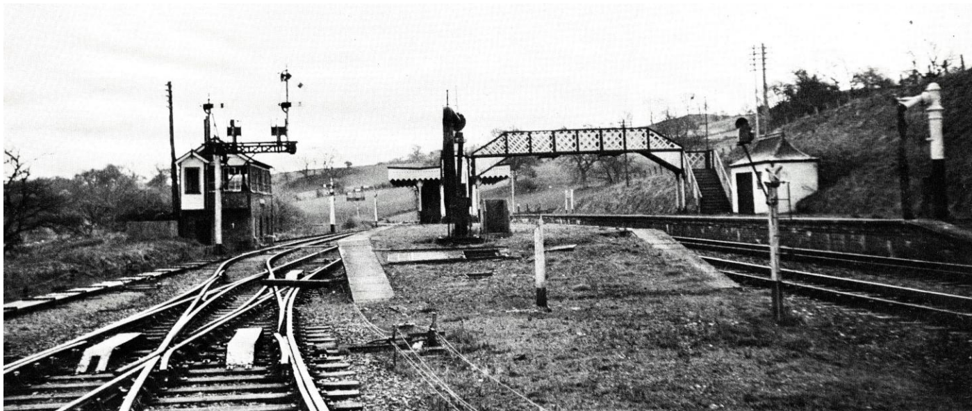
View eastwards, May 1967. Only the demolition train has yet to call. Despite nominally independent origins, everything here is pure GWR. Photograph: K. A. Jagers.
