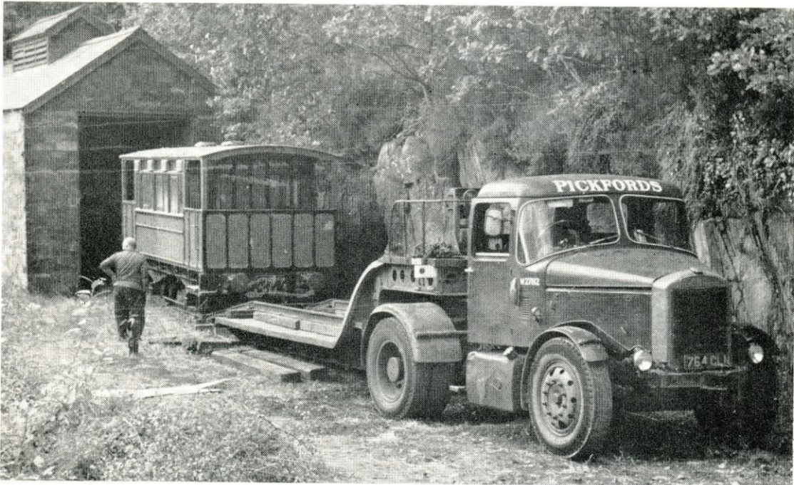
Before the removal of "Fire Queen", a four-wheel directors saloon from the Padarn Railway was taken from another shed at Dinorwic Quarry to Penrhyn Castle, where it will be exhibited with "Fire Queen"
