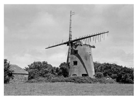
It was in a complete condition in 1934 when the Royal Commission of Ancient Monuments survey recorded it in great detail with a photograph and drawings. The tower is 30 ft 6 in high and has a diameter of 19 ft 6 in at the base; the span of the sails was 69 ft 6 in. On the top of the tower a timber curb carried an irongeared rack upon which the cap was rotated to turn the sails into the wind, by means of an 8 ft diameter chain wheel.
