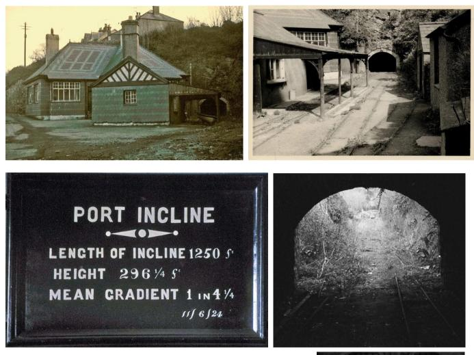
Inside the tunnel, as seen here the dual 2 ft gauge line started to rise on a 1 in 4 inclined plane, later crossing the Caernarfon railway on its way up the hillside.
