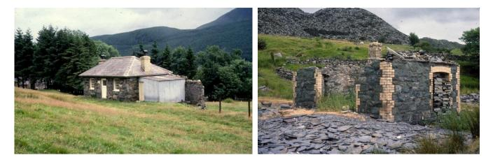
The extensive workings of Glanrafon Slate Quarries were connected to the main railway by an incline that descends on the north side. The ruined building at the foot was a weighbridge (573640;
