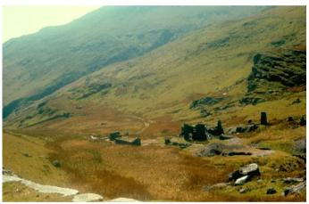
The isolated slate working on the west side of the valley opposite the Prince of Wales mill was that of Dol-Ifan-Gethin quarry, also with an incline and water-powered dressing mill. It was not connected to the tramway, instead sending its products by cart down the valley road.
