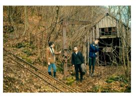
The more prominent remains in the vicinity of the incline, a crushing mill, workshop with hand crane (above right), and the drum house itself higher up, are from a much later working for granite. A tramway may be followed from the incline head for a short distance southwards along the hillside to the Gwydyr Quarry, in which track and points survive amongst the young trees.
