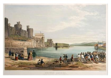
At Conwy, the "Medieval" stone towers were presumably an attempt to appease those objecting to the intrusion of the railway into the environs of the Castle. These towers, of Mona marble, support the twin tubes carrying the railway lines, each 400 ft long and weighing 1300 tons. On the inland side of the
