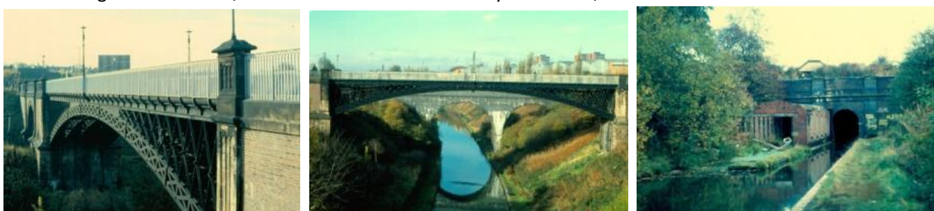
Galton Bridge at Smethwick, and the west entrance to Gosty Hill tunnel, near Old Hill.....
